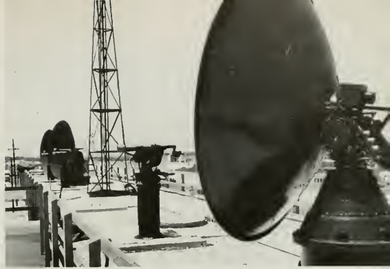
4. Huge radars at launching site begin tracking the missile, then as it moves down-range each station in turn takes over.
